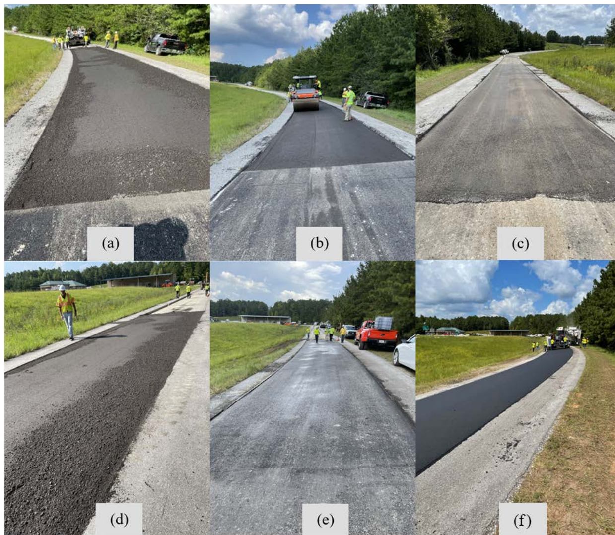
FIGURE 4 Paved CCPR Sections on off-ramp; (a) foamed asphalt with active filler, (b) engineered emulsion, (c) CR rejuvenator, (d) emulsified bio-based rejuvenator; (e) emulsified bio-based rejuvenator, and (f) HMA thinlay overlay.
