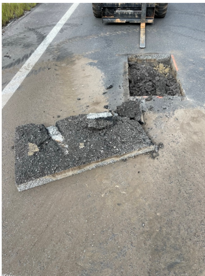
FIGURE 7 Material collection for mix design of 3 rd generation re-recycled CCPR.
