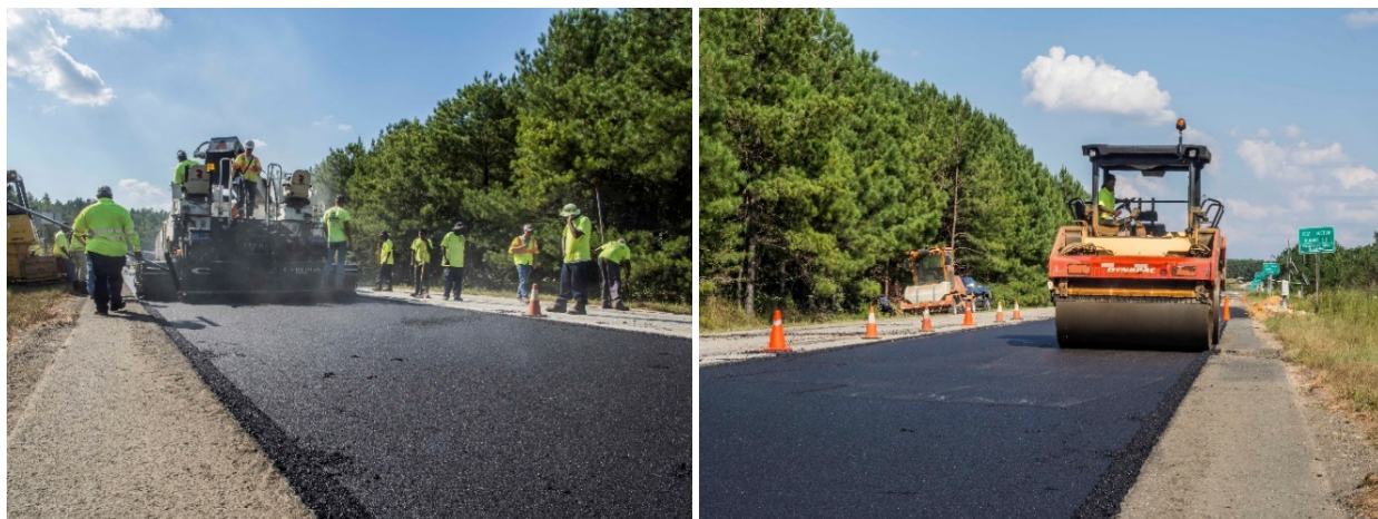
FIGURE 3 Laydown and compaction of S1 base mix.
