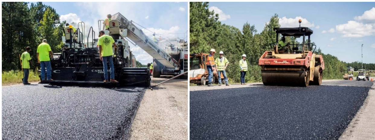
FIGURE 4 Constructing Section S10 with a BMD mix.
