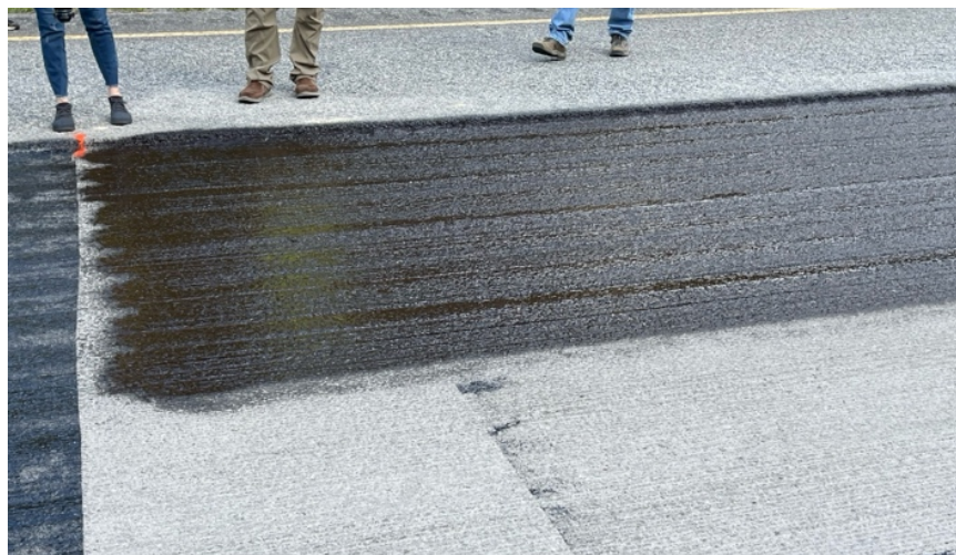
FIGURE 3 Tack coat application after milling in Section W4.
