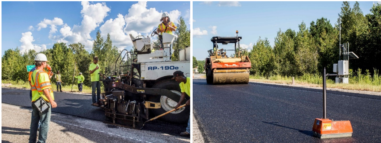
FIGURE 5 Constructing Section S11 with a volumetric mix.
