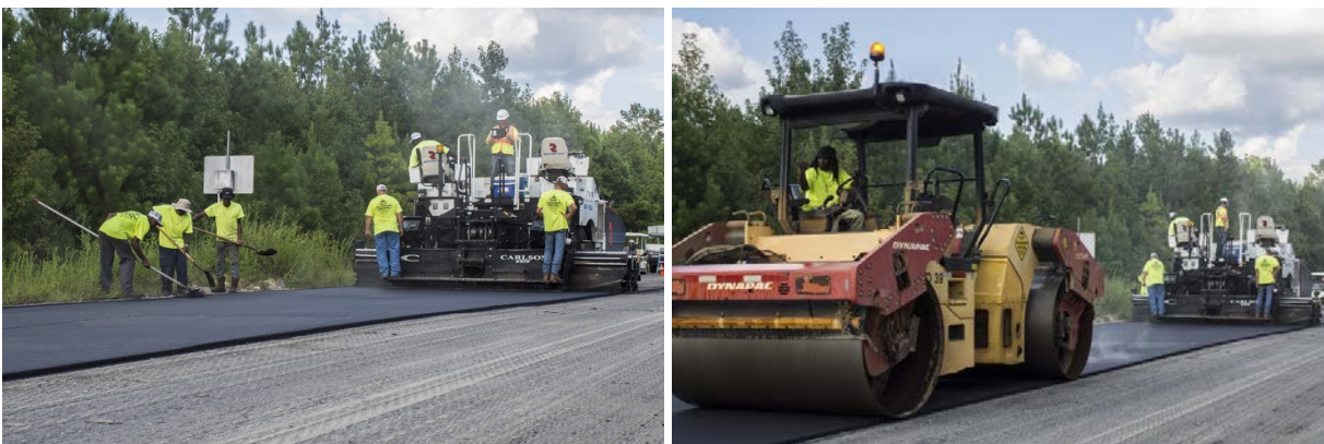
FIGURE 1 N10 mix placement and compaction.
