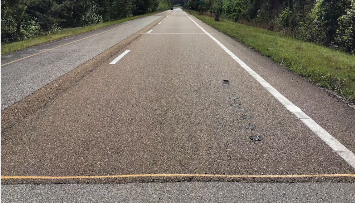
FIGURE 3. Test Section S2 after completion of second trafficking cycle.
