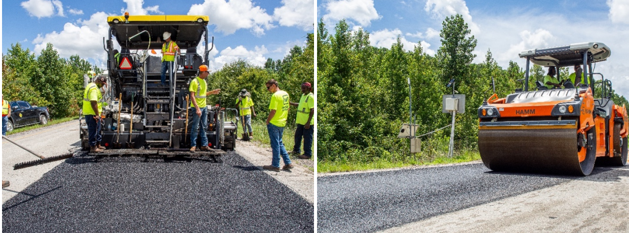
FIGURE 5 Construction of Section S7A.
