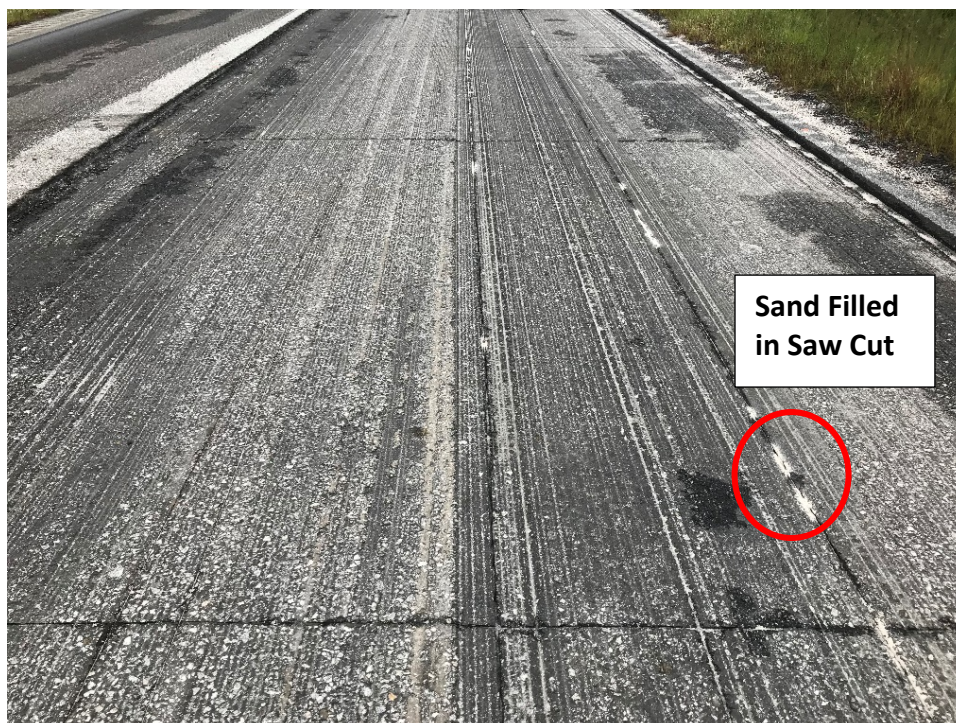
FIGURE 1 Deep saw cuts to simulate pavement cracks.
