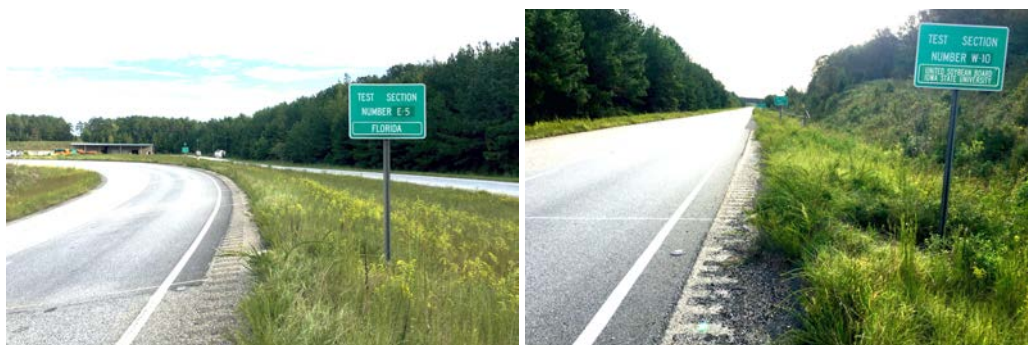
FIGURE 2 Paving of Sections E5A and W10.
