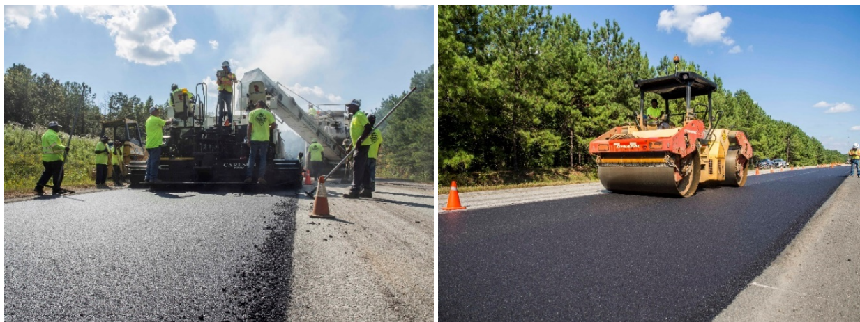
FIGURE 4 Laydown and compaction of S1 surface mix.
