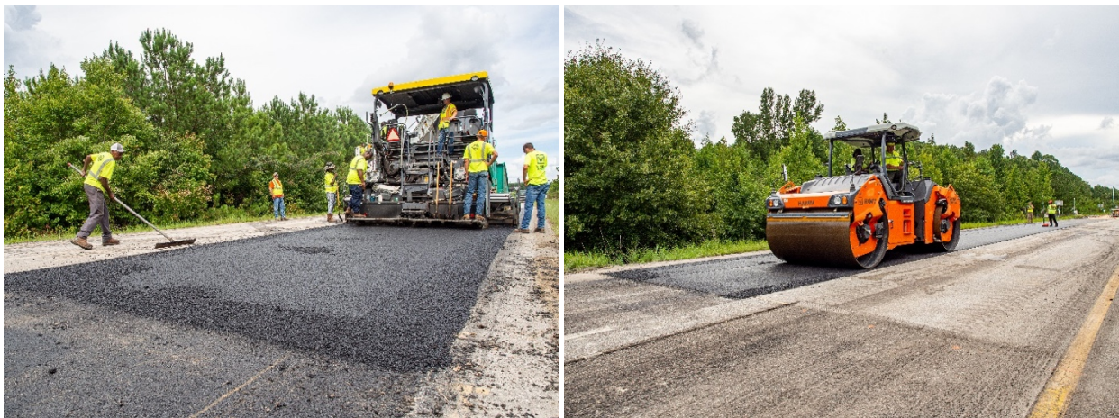
FIGURE 6 Construction of Section S7B.
