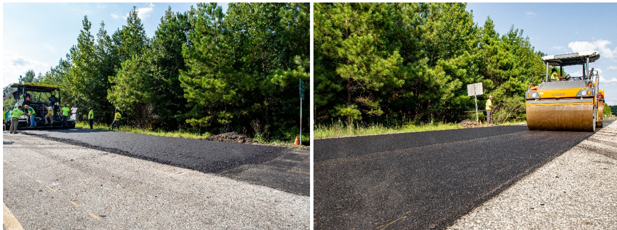
FIGURE 16 Laydown and compaction of N9 surface mix.
