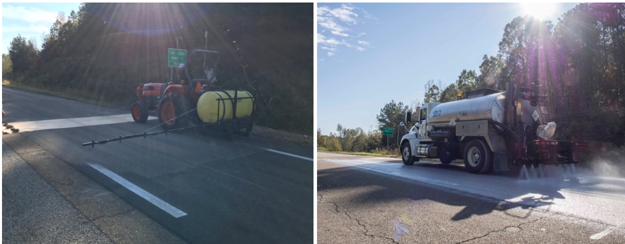
FIGURE 1 S3-A and S3-B application of spray-on rejuvenators.
