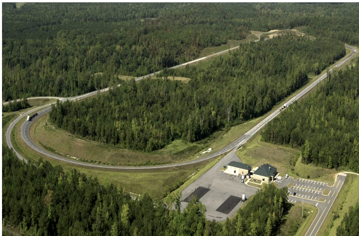
FIGURE 1 Aerial photograph of the NCAT Test Track.
