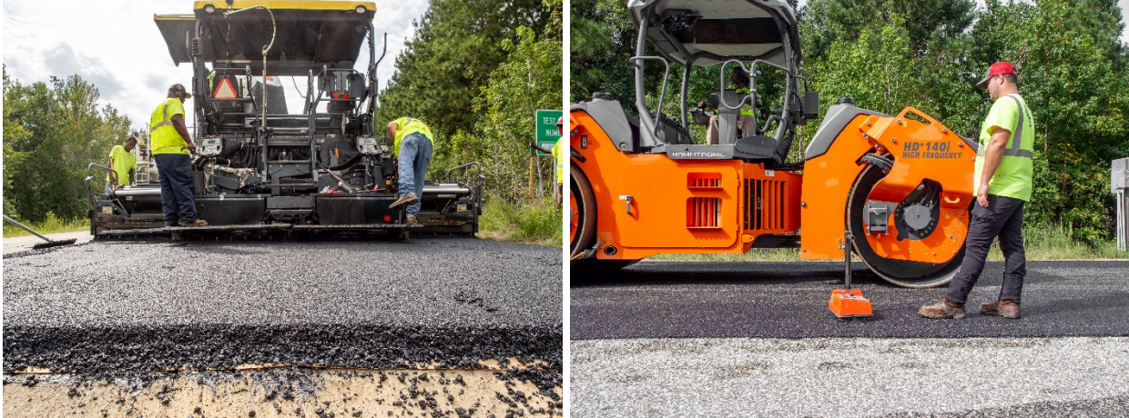
FIGURE 6 Constructing Section N6 with a BMD mix.
