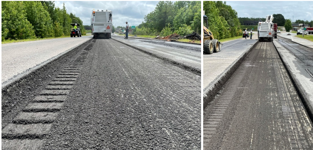
FIGURE 2 SMA and dense graded asphalt layer milling (left) and CCPR layer milling (right).
