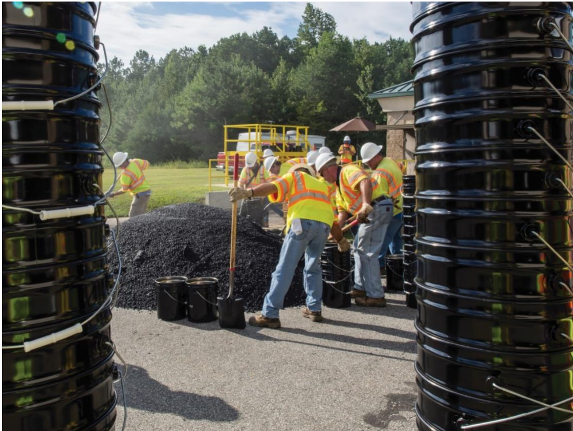
Figure 2. Mixture Stockpile Sampling
