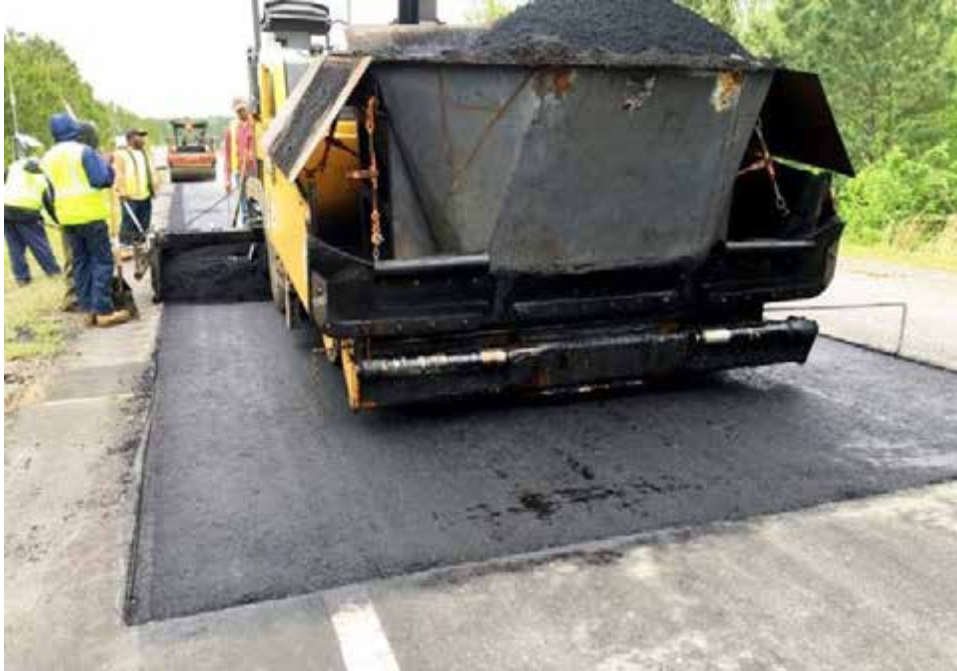
Figure 2 First Repave of Section N7
