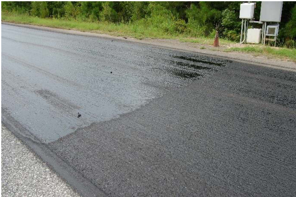
Figure 3 Transition Between Low and High Tack Application Rates in Section N9
