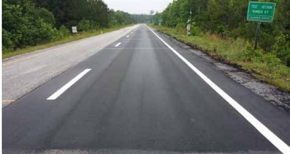
Figure 7 Section N7 After the Second Repave
