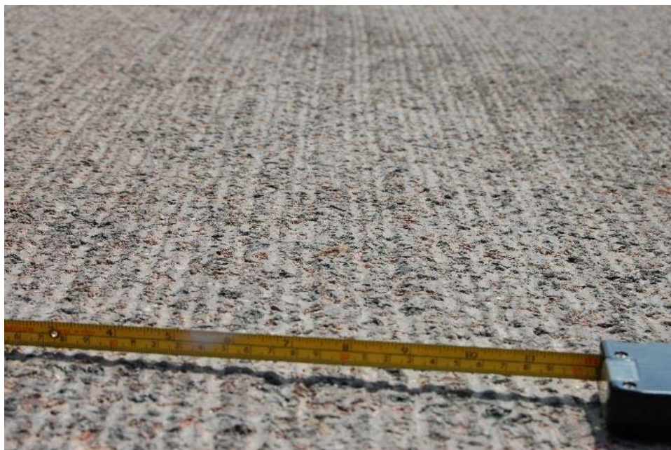
Figure 1 Finished Micro-Milled Surface of Section N9
