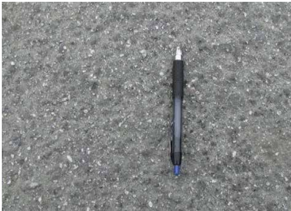
Figure 2 Surface Treatment Layer with Sand Seal
