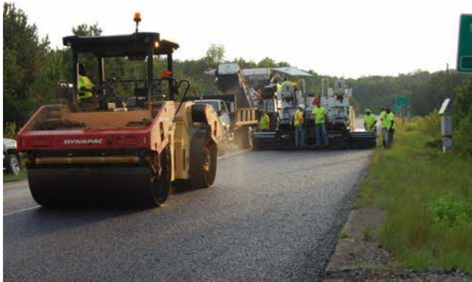
Figure 2 Paving a Test Section for the 2015-2017 Research Cycle
