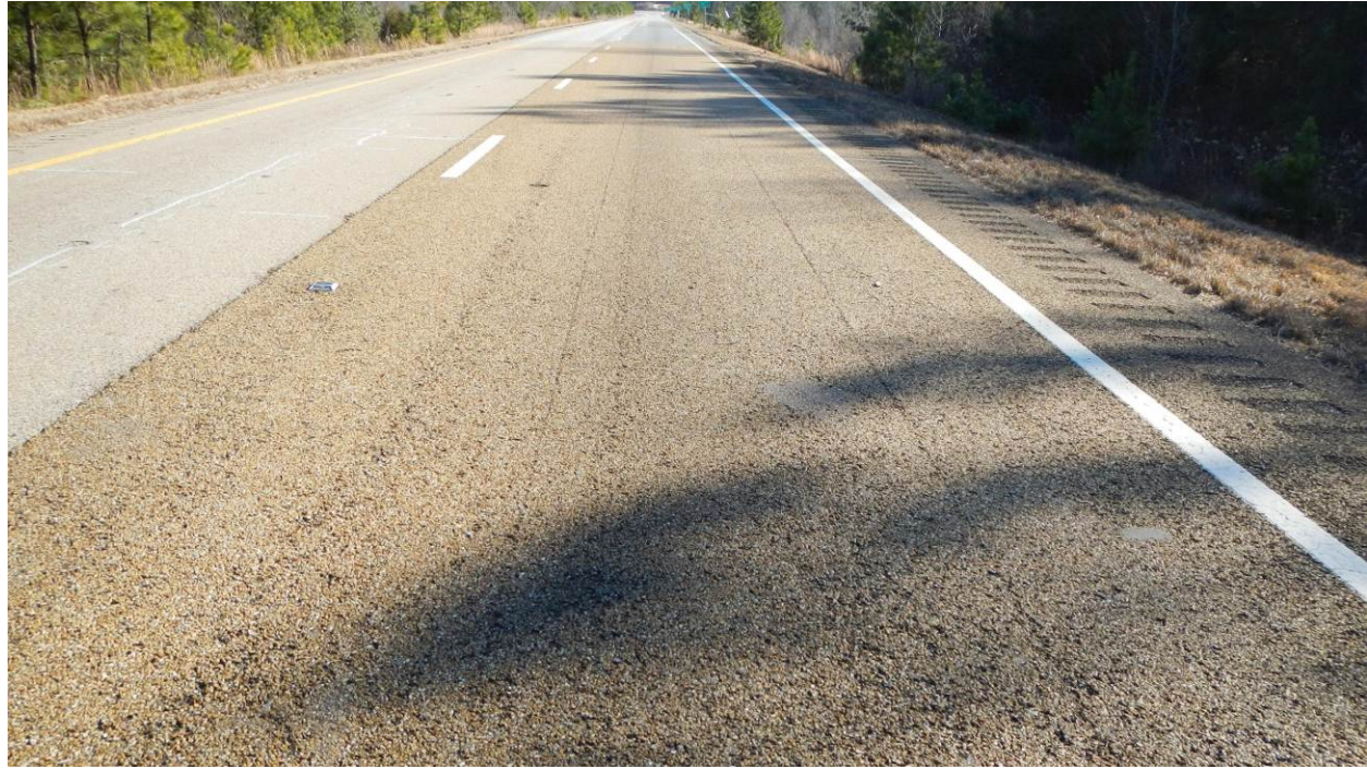
Figure 2.6 Photograph of the Mississippi Gravel OGFC Section Beyond the Transition Area
