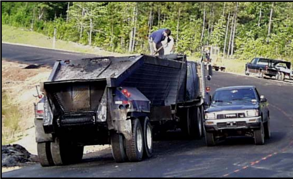
Figure 3. Removing Shovel Sample from Truck on Roadway
