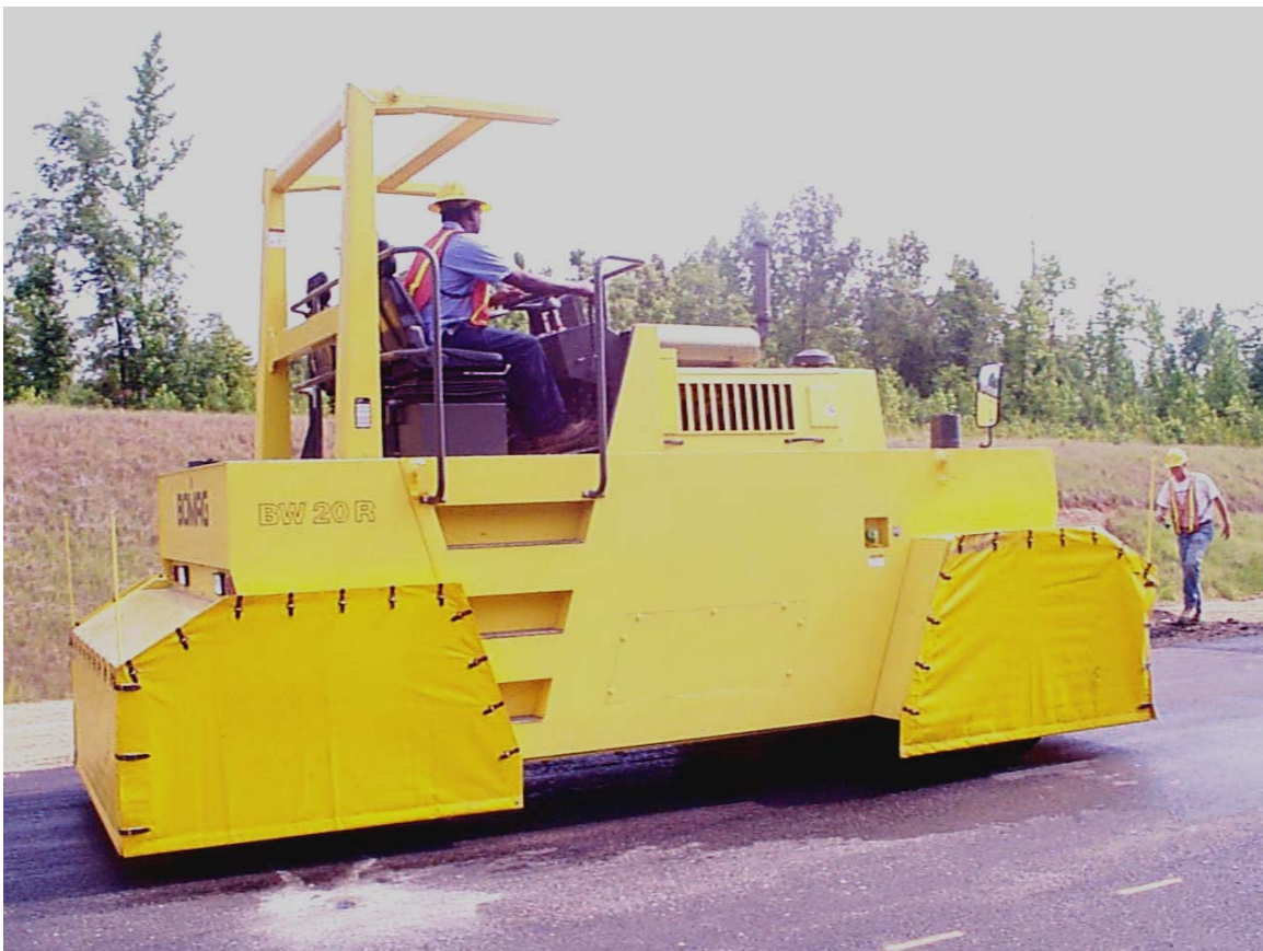
Figure 9. Pneumatic Rubber Tired Roller Compacting Track Mix
