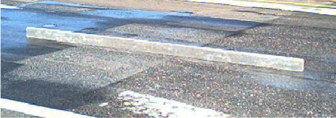
Figure 24. Typical Ground Joint Texture
