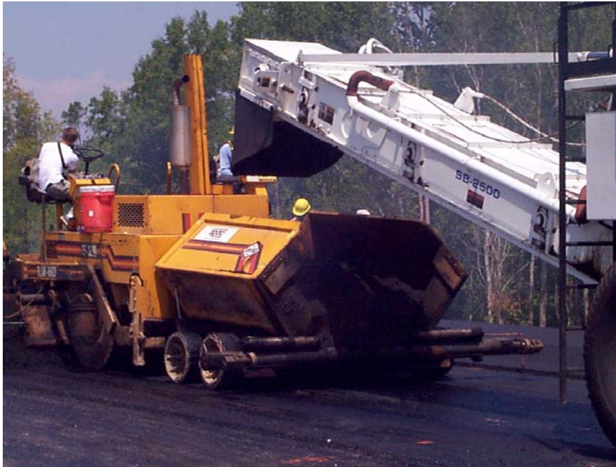
Figure 6. Conventional Paver Placing Experimental Mix on Track
