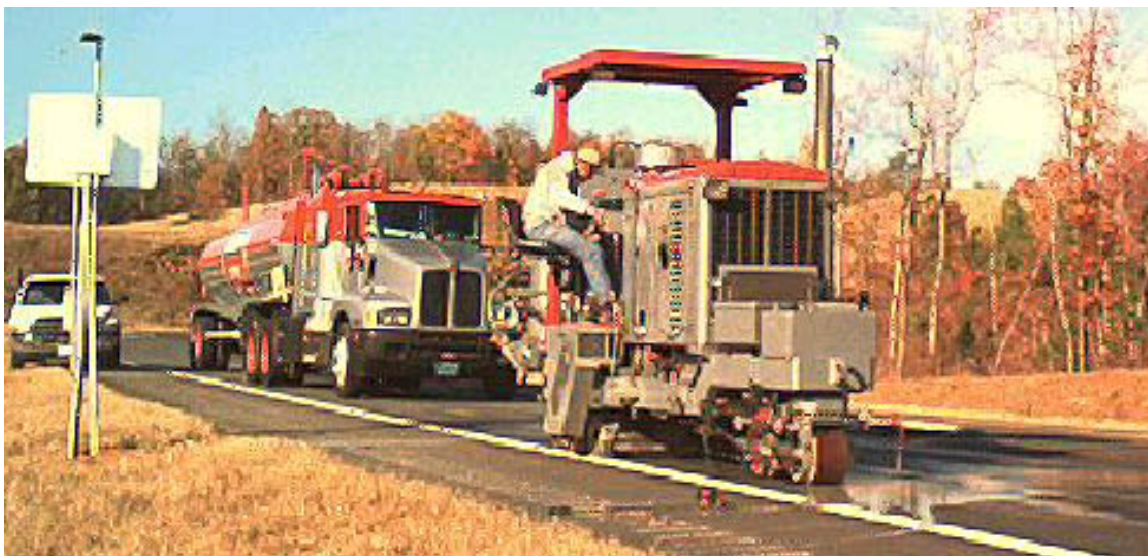
Figure 22. Typical Diamond Grinding Operation
