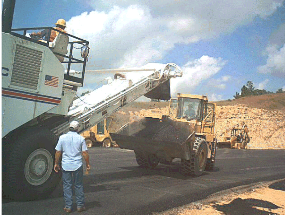
Figure 10. Sampling Research Mix by Dumping into Front End Loader
