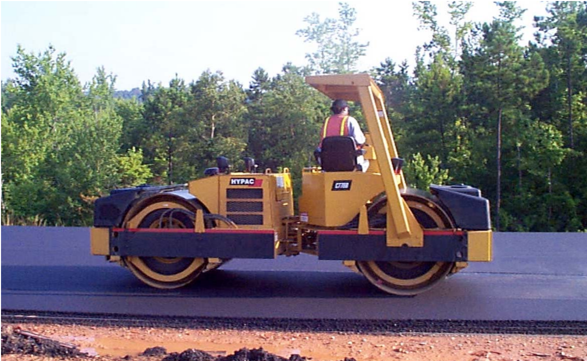
Figure 8. Vibratory Steel Wheel Roller Compacting Track Mix
