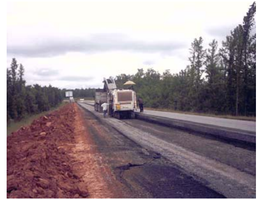
Test Track reconstruction in progress for installing eight structural test sections (2003).
