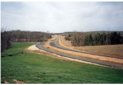
NCAT Test Track after HMA base course paving (2000).
